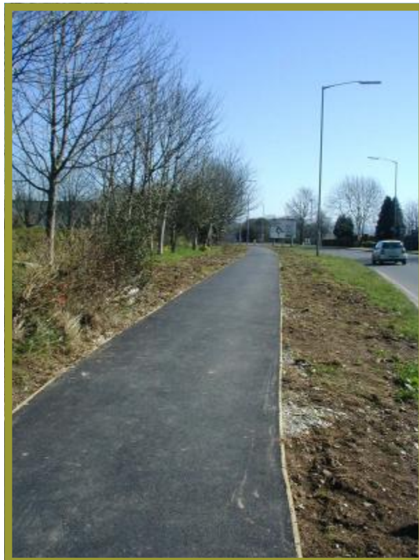
Right. Near Granite Way is the start of the new footpath/cycleway to Kit Hill
